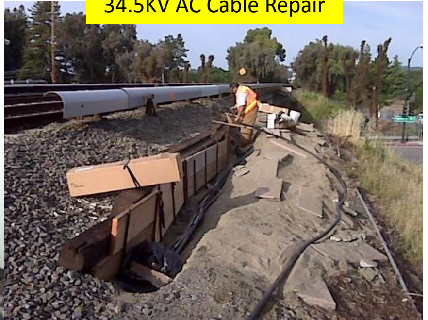
34.5KV AC Cable Fault
